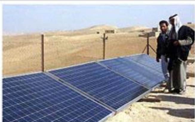
Inspecting part of the new school solar array is Mr. Mahmoud Al-Magada (left). He commented that this solar power plant is the fulfillment of a great dream held by the Village Council for leaping into the 21st Century at full speed.
