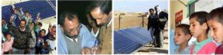
Photos taken on the day of installation. Click on the photos to see detail, and get reproduction-quality images.
