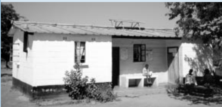
Figure I.3. Photovoltaic system supplies power for a vaccine refrigerator and lights at a health clinic in Zambia.
